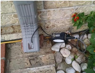
Continuity between the rain gutter sections was checked before beginning this project since some rain gutters are not metal. This rain gutter was painted to match the house trim, so continuity between sections was an initial concern.
